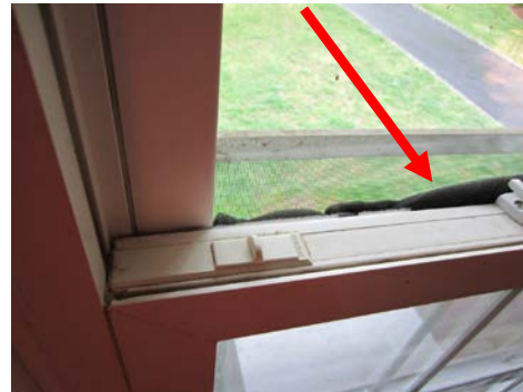
Accessory compressible foam gasket (installed)
